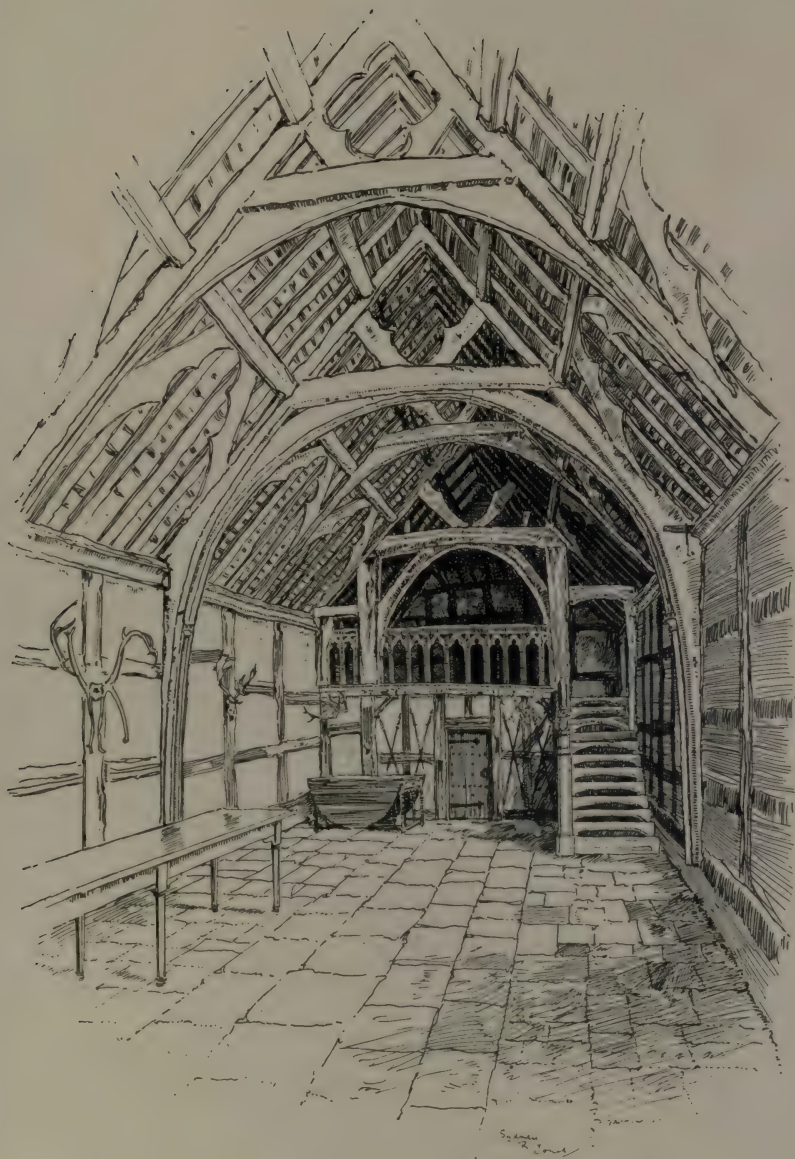
INTERIOR OF THE HALL, LOWER BROCKHAMPTON, HEREFORDSHIRE
